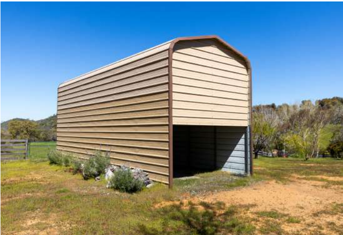
RV Storage Building: 12' x 31' consisting of 372 square feet; power and lighting
