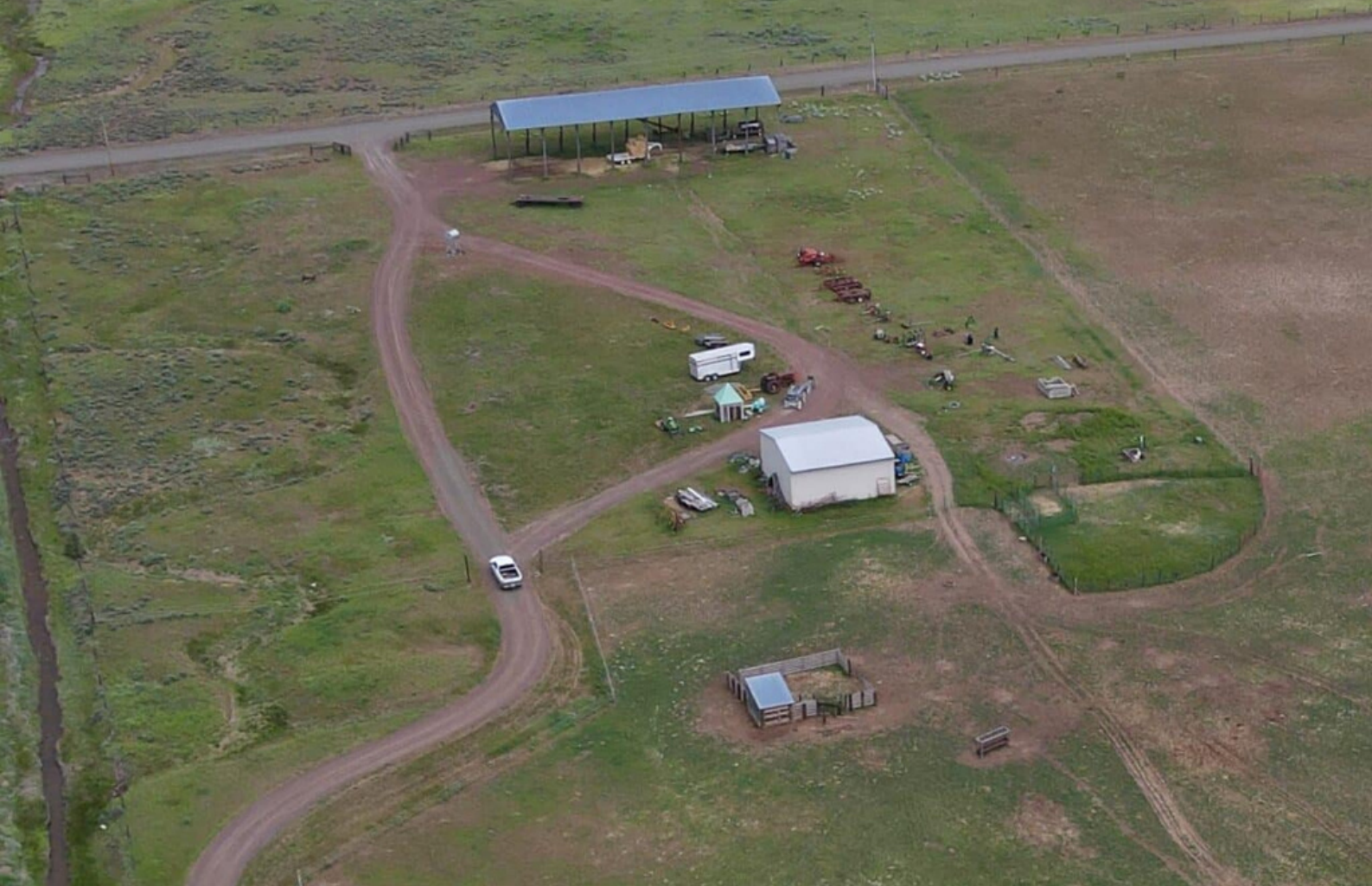
35x35 metal shop at the property entry
