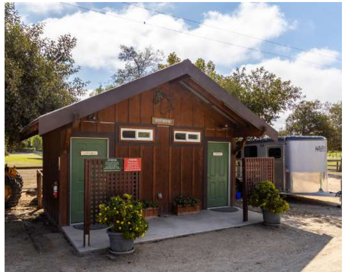
Pictured Above: Restrooms
