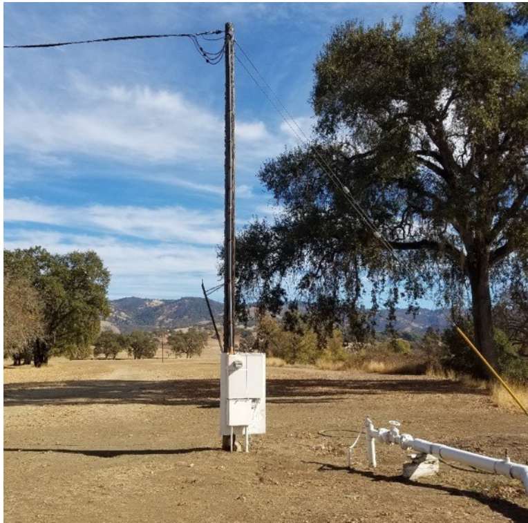
Photo 33, Location 23: Power box for water pump to irrigate field.
