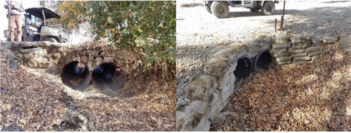
Photo 31 and Photo 32, Location 22: Culvert and road over drainage that feeds into Mewhinney Creek.
