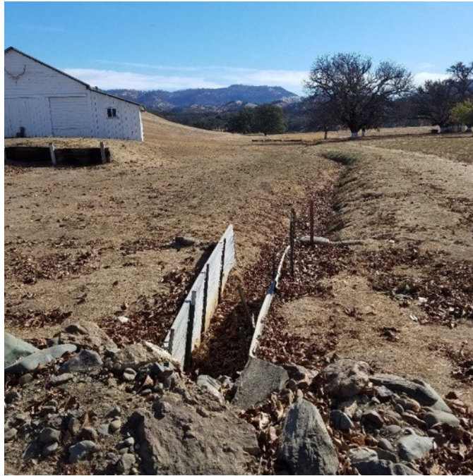
Photo 19, Location 14: Drainage ditch to collect and divert water from barns and residence.
