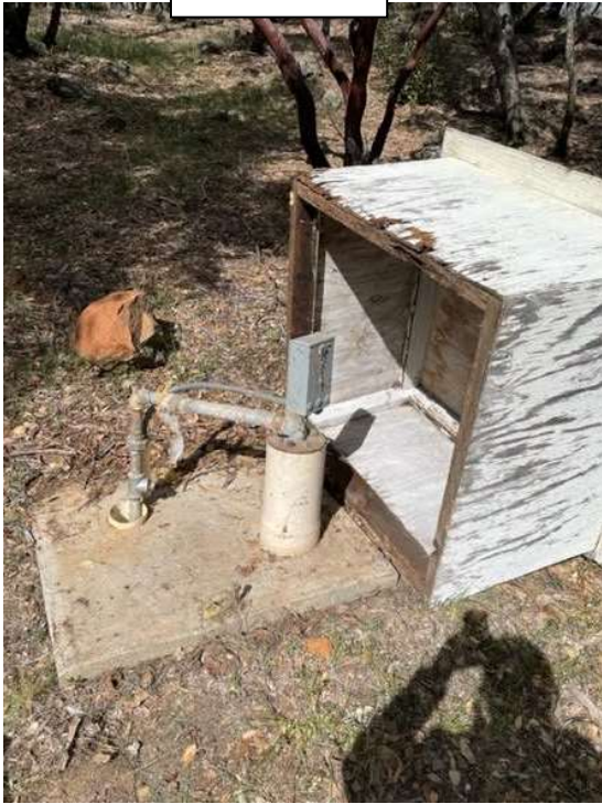
Booster Pump & Pressure tank
